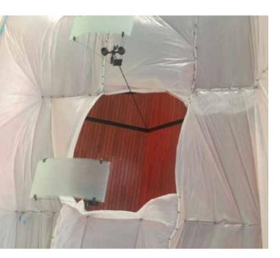
Because the original wood was custom-designed and installed by specially trained artisans, removing or replacing the wood did not seem to be a good option for the convention center. The client ultimately chose to have a tape-and-seal fumigation performed.
