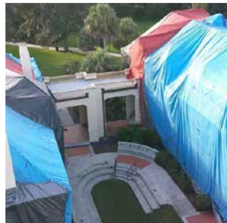
The Thomas Center is carefully tented during its fumigation by Southern Fumigation.
