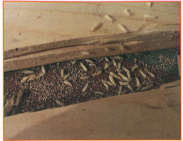
Drywood termites and fecal pellets in a gallery. The pellets have different colors, even though the wood is only one color.
