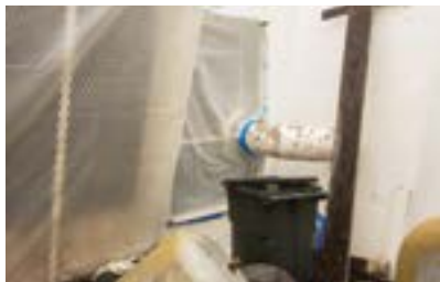
The vessel was taped-and-sealed.
